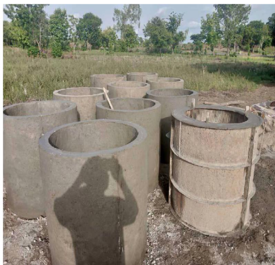
Preparatory work for a community potable water well project in Tchikawa, Binah Prefecture (May 2024).
